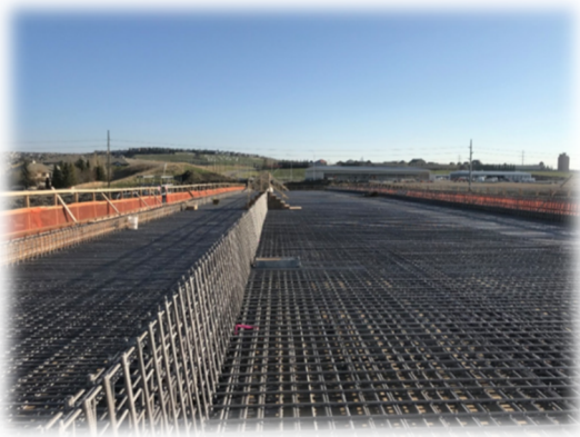
Bridge 41 ready for concrete
