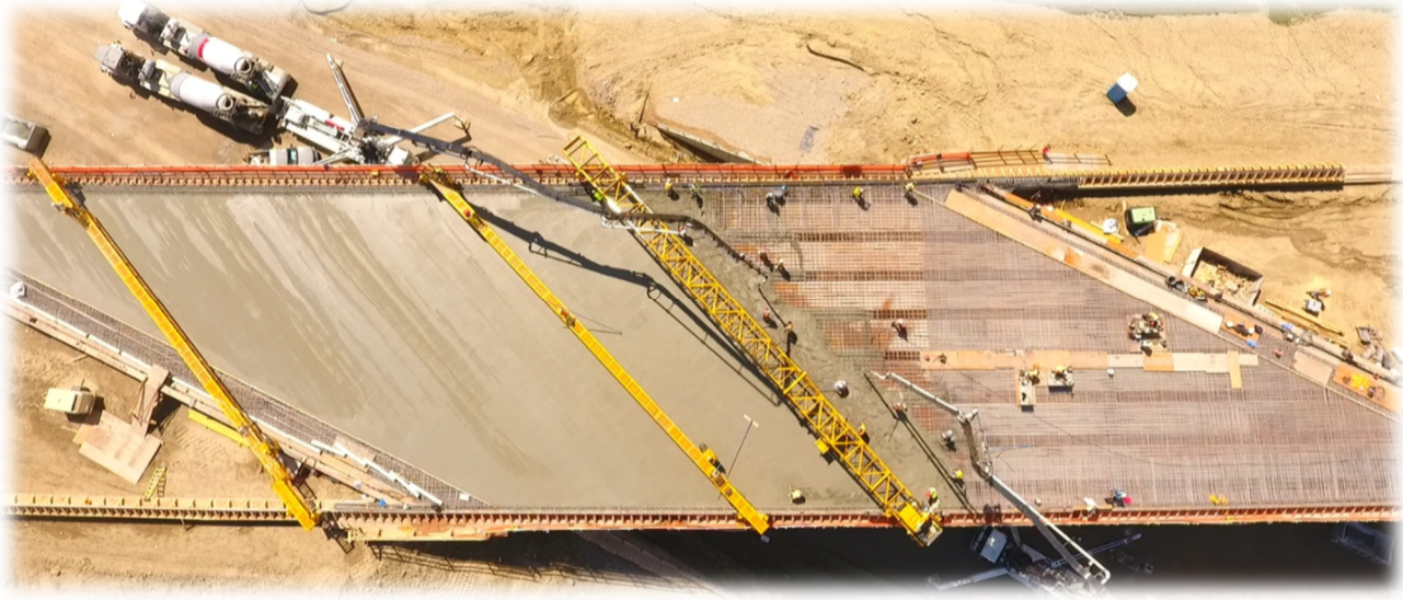
Bridge 19 Deck Pour, the final project bridge deck pour.
