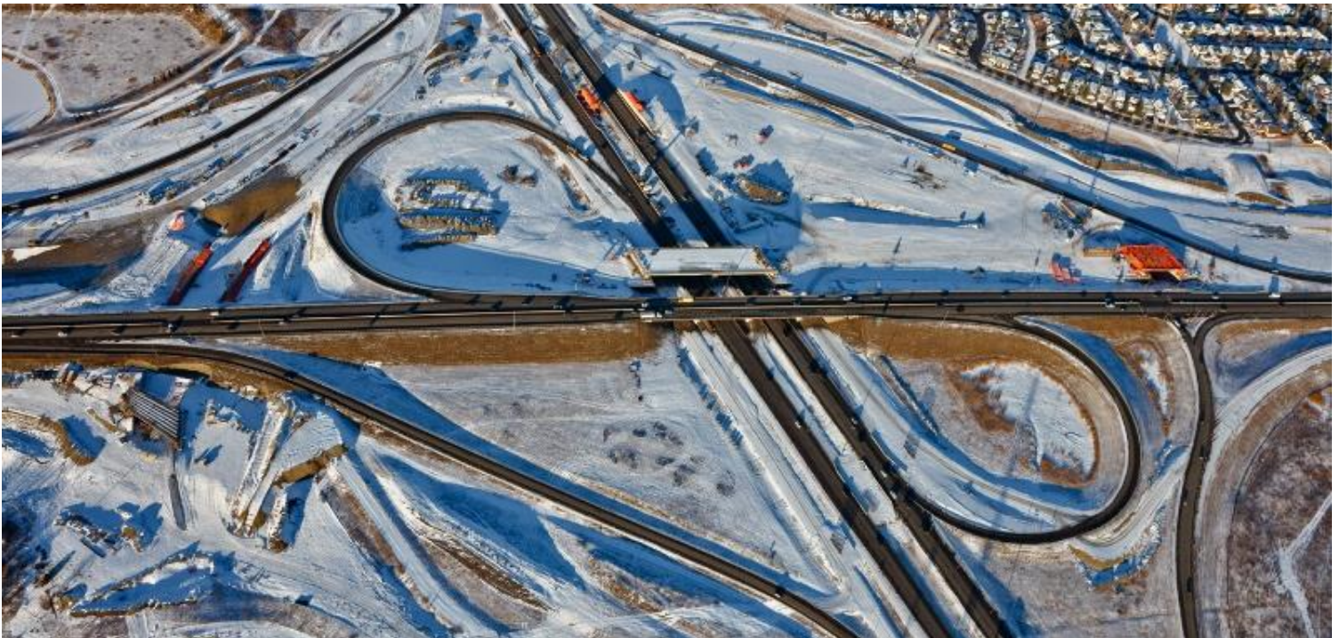
Bridges taking shape in the Macleod Trail interchange
